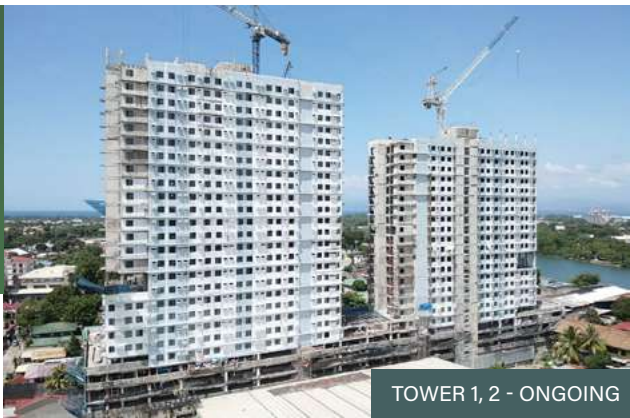
Casa Mira Towers CDO | 6,315 m 2 Brgy. Kauswagan, Cagayan de Oro City | CDO Tower 1 = 542 units | Tower 2 = 444 units
